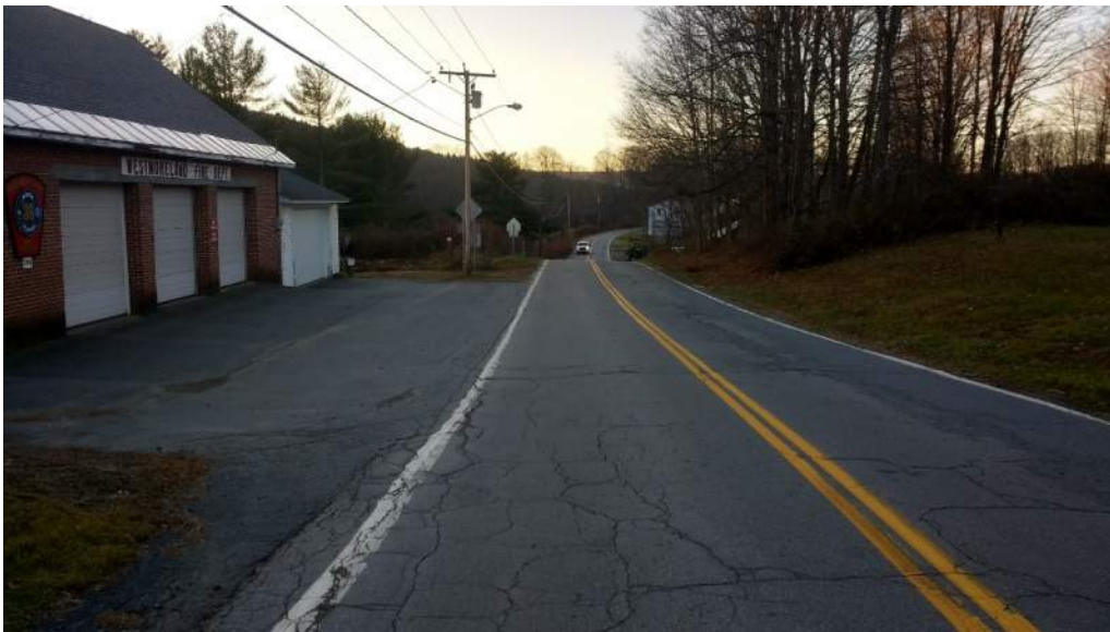
Apron at front of station.
